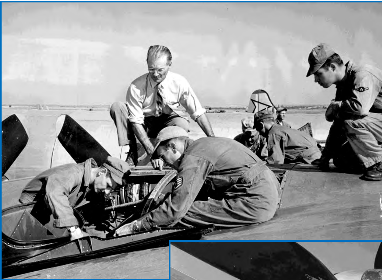
Top: Air Force enlisted maintenance technicians perform hands-on training for the Pratt & Whitney R-4360 engines in the B-36.
