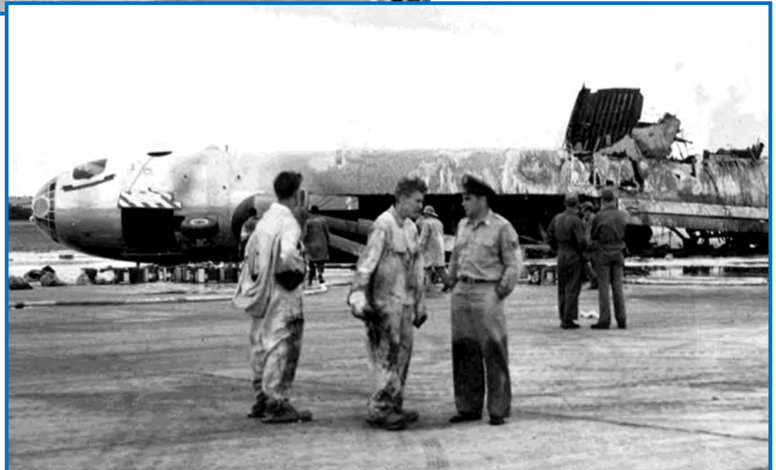
Above and Right: When B-36F (50-1066) crashed during a training mission from Carswell AFB on May 28, 1952, it took dozens of firefighters to put out the blaze. A loose engine panel caused the pilot to attempt a heavy weight landing when the landing gear broke and the aircraft skidded down the runway and burned.
