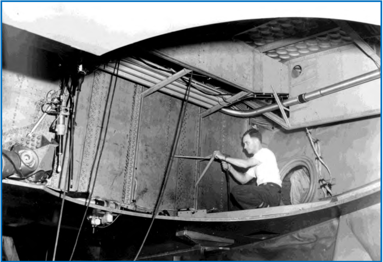
Top: Technician working inside the spacious wheel well of the XB-36.
