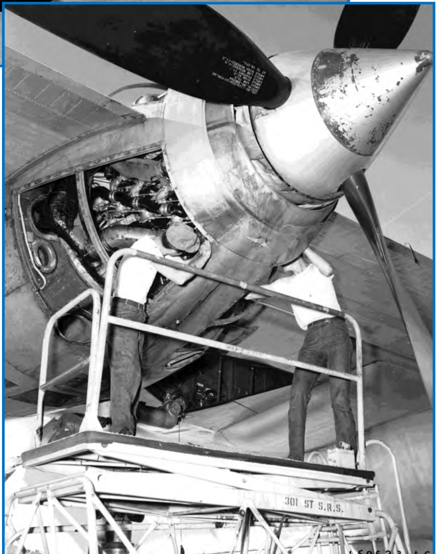
Right: Large access panels allowed maintainers easier access to the engines on the B-36. Tunnels running inside the wing allowed for limited access to the engines in order to perform in-flight maintenance during long endurance missions.
